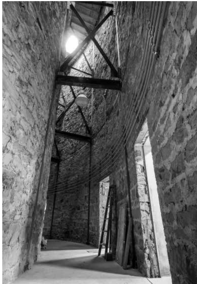
Interior stonework and steel frame of bandshell.
